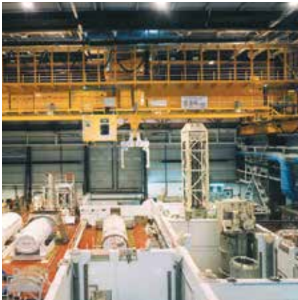
Wellman Booth nuclear fuel and waste handling.
