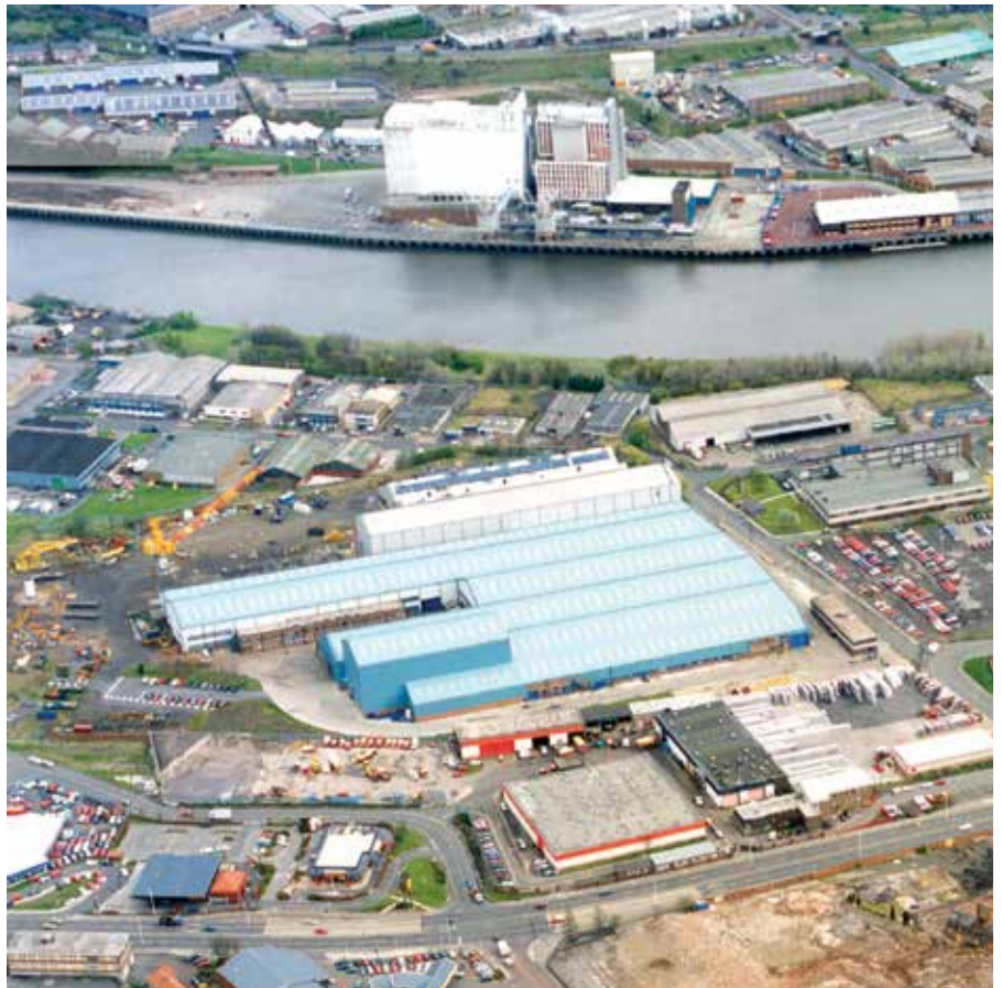
Clarke Chapman group headquarters, Gateshead, Tyne & Wear, England.
