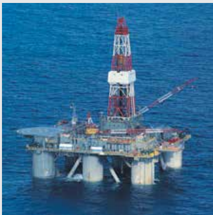
Typical Stothert & Pitt offshore installation.
