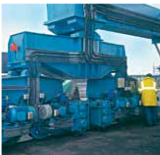
Onsite electrical control system installation.
