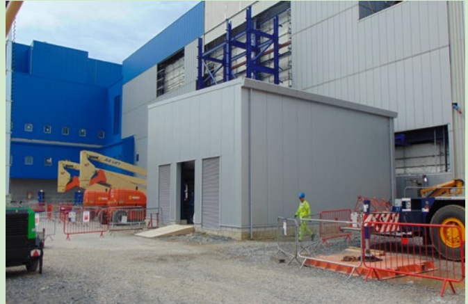
Inside the Compressor House
