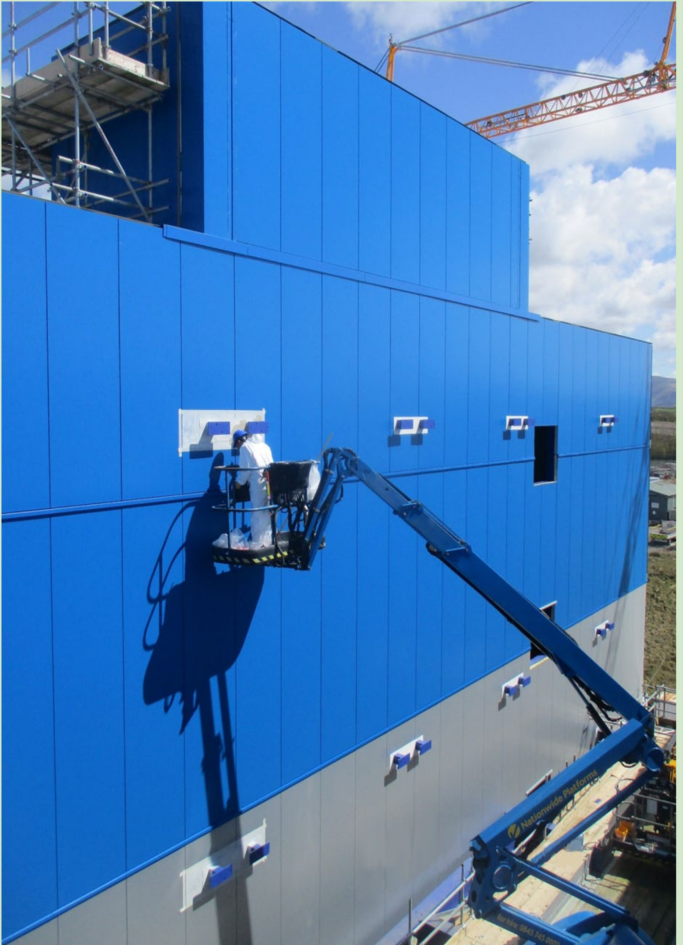
Cladding, progress on the rear of the Grout Plant.
