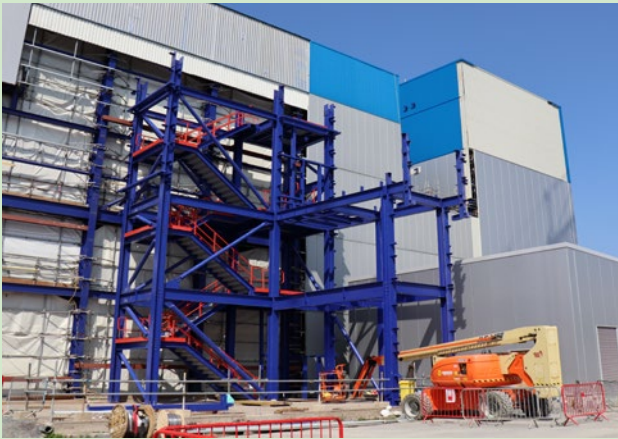
RRRB Steel Erection – Final staircase module
