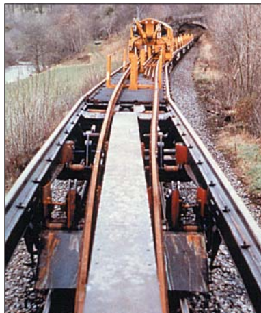
Long welded rail train laying rail
