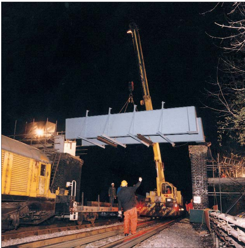
12 tonne general purpose placing a bridge section. Railtrack
