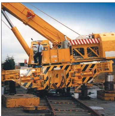
75 tonne crane undergoing test.
