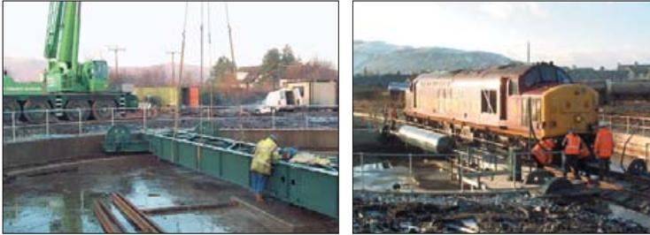
Removal from Marylebone Station, London of a turntable used to turn steam locomotives. Complete rebuild and refurbishment undertaken and was transported to Fort William and installed in new foundation pit. The Turntable was originally built in 1937 by Cowans Sheldon. Heritage funded.
