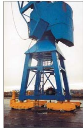
Manufacture and install a new portal legs assembly to 10 ton DD2 quayside crane after the crane had been damaged.
