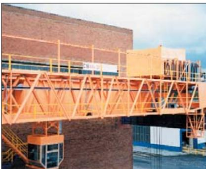
Corus: This overhead crane was dismantled from a redundant steel works, modified to suit new span and relocated and installed at another plant.
