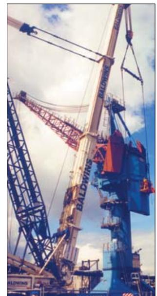
The installation of a replacement slew ring on a Butterley quayside crane carried out by using the largest telescopic mobile crane in the UK.
