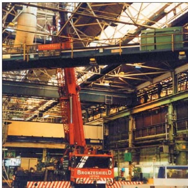
Ford Motors: To dismantle and modify span and relocate within the factory, two 20 ton electric overhead travelling cranes.
