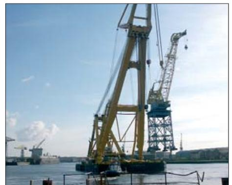
Relocation of a dockside crane using the "Asian Hercules II" on the River Tyne. Client A&P Tyne
